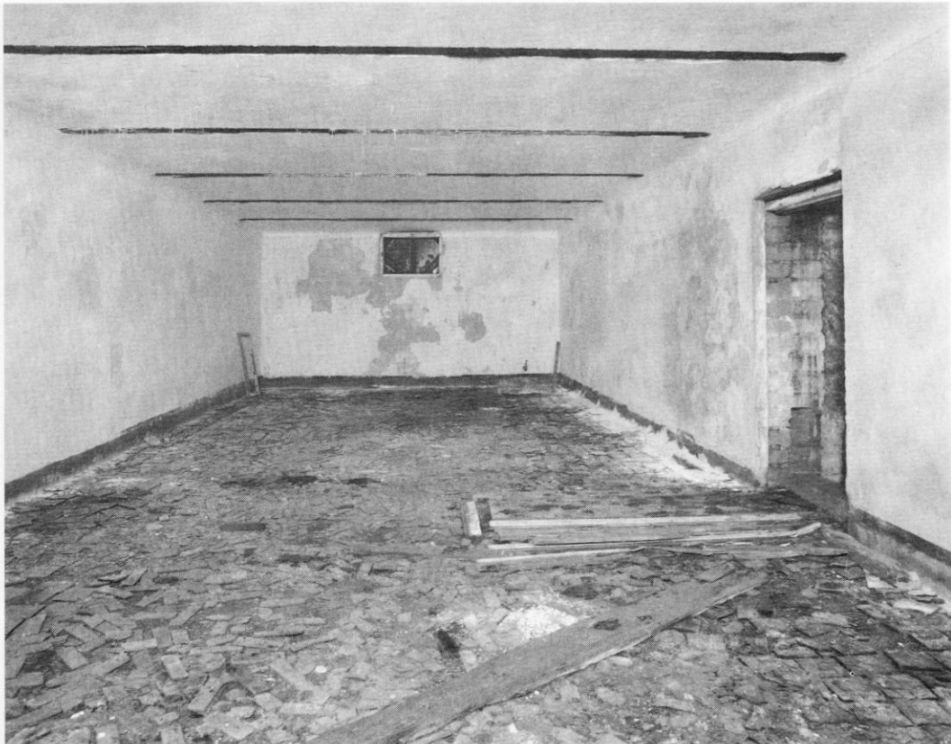
The main living quarters photo by Nick Catford
